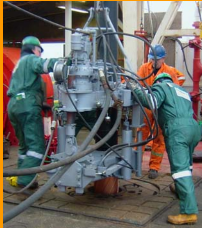
The Franks Casing Crew gets stuck-in, thanks guys.
